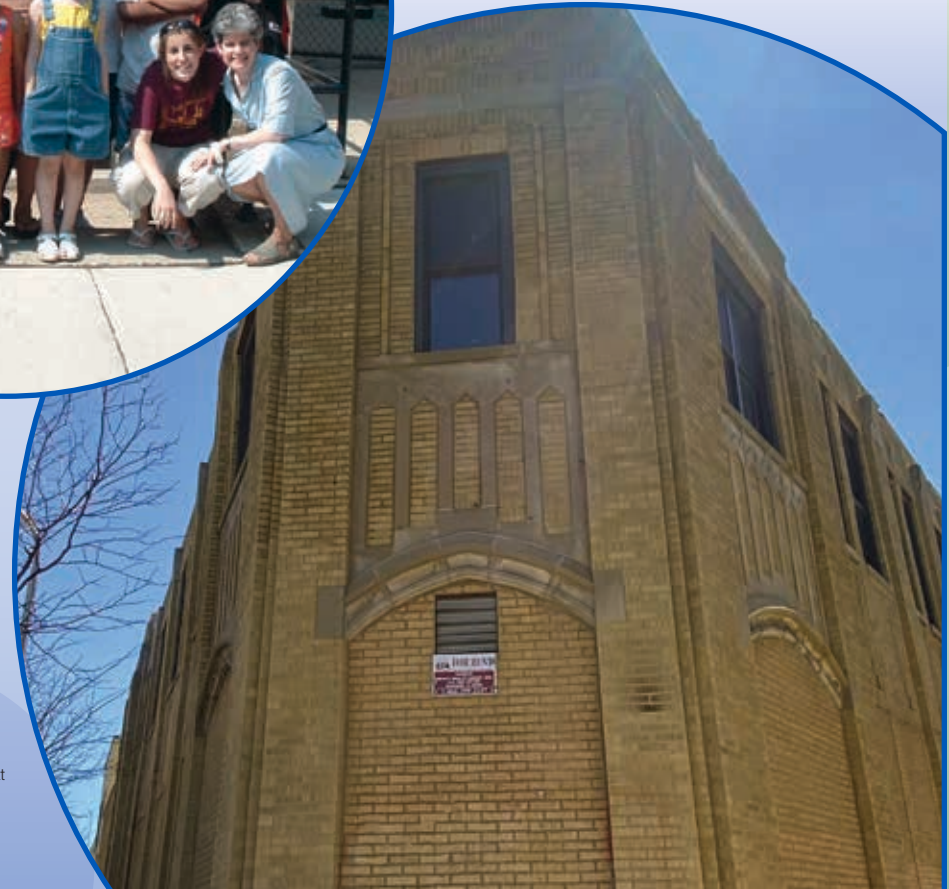
Site of new administrative offices and programming for West Humboldt Park at 4123 W. Grand Ave.
